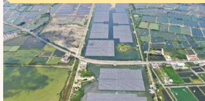
Chiayi Xinwen Detention Basin 36 MW
