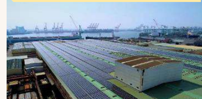
Kaohsiung CSBC Corporation 13.8 MW
