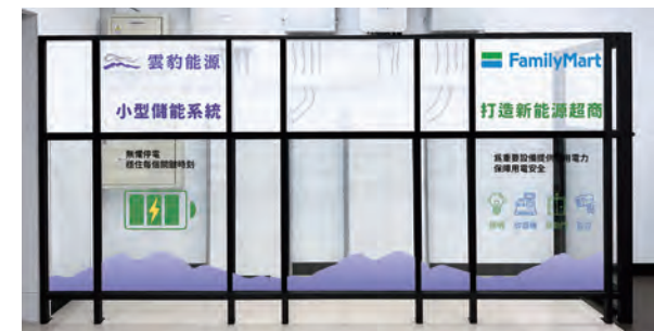
Small-scale Energy Storage Equipment Installed at the FamilyMart Neihsu Store in Hsinchu.
