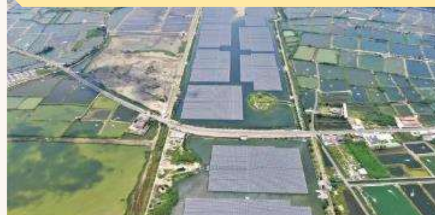
Chiayi Xinwen Detention Basin 36 MW
