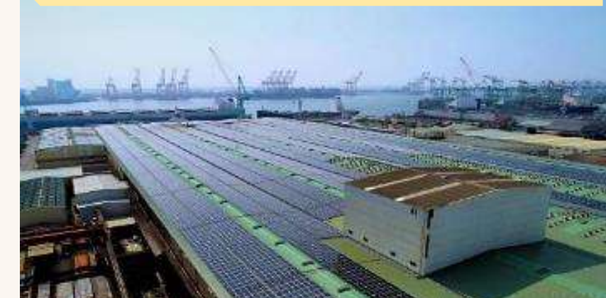
Kaohsiung CSBC Corporation 13.8 MW
